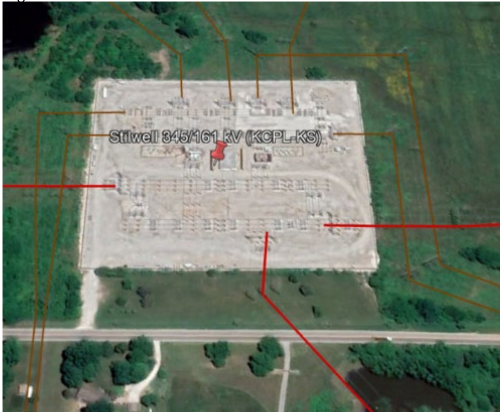
Figure 28 – Stilwell 345 kV substation
