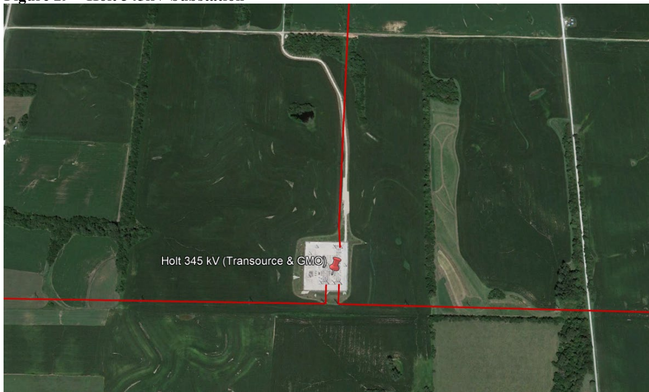
Figure 29 – Holt 345kV Substation
